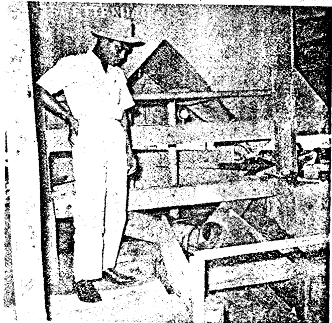
General view of the hydrocyclone plant, showing header box and five gravity feed pipes, two of which are in use
