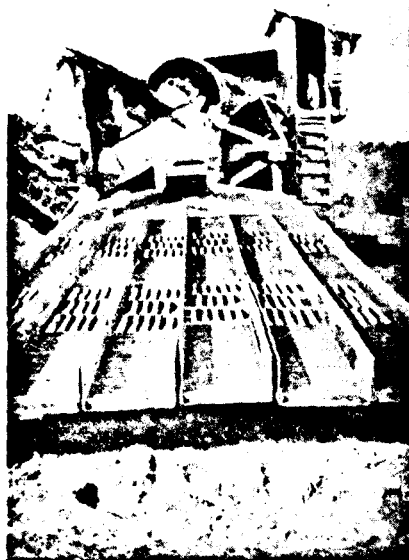
Arrangement of sluice boxes and riffles at the property of the Ferey Mining Company, in White County, Ga.
